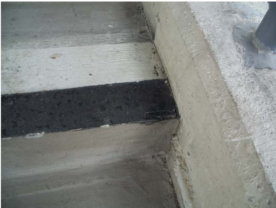
Photo #7 – Stair Nosing
